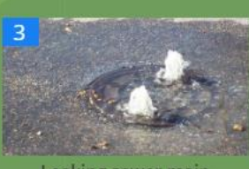
Leaking sewer main
