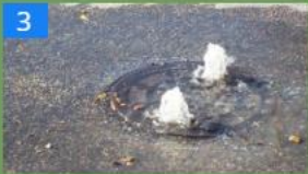
Leaking sewer main
