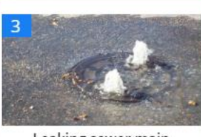
Leaking sewer main
