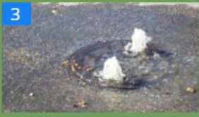
Leaking sewer main
