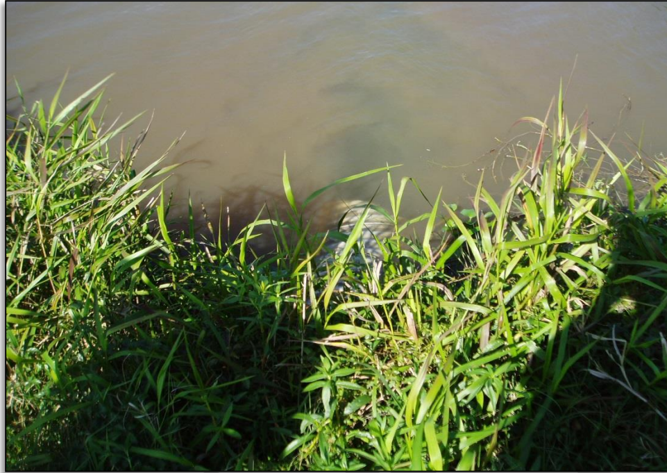
Figure 7-5 Straight pipe discharge East Fork
